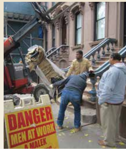
Before, during, and after the newel post replacement at 6 South Portland Avenue in Fort Greene, Brooklyn.
