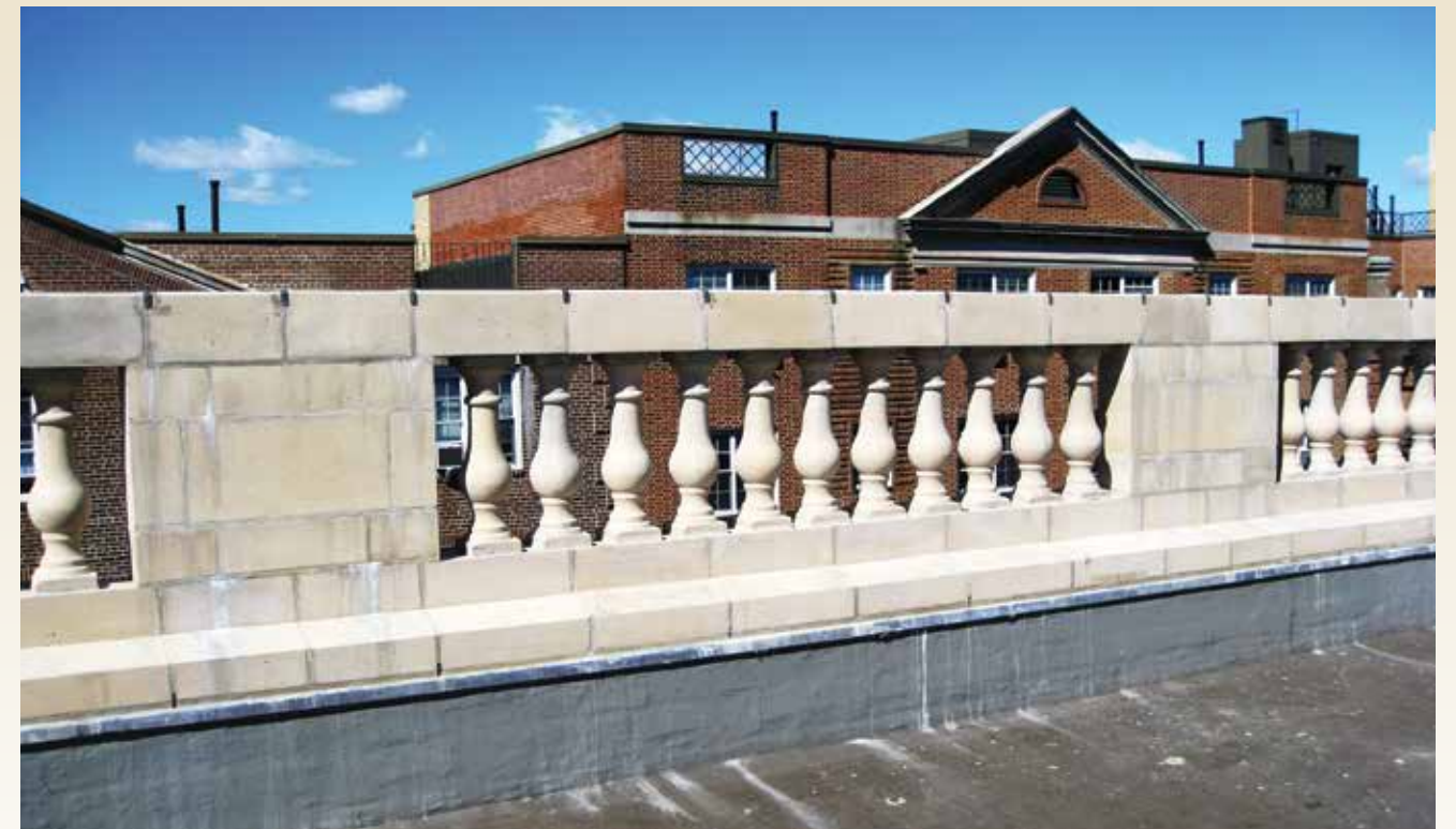
Cornice repair work in the Jackson Heights Historic District.
